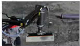
■ Effortless kerb lifting & placement
